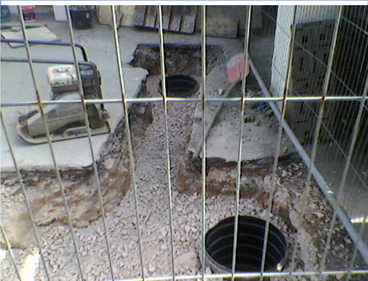
Work in progress at St Bede's School
