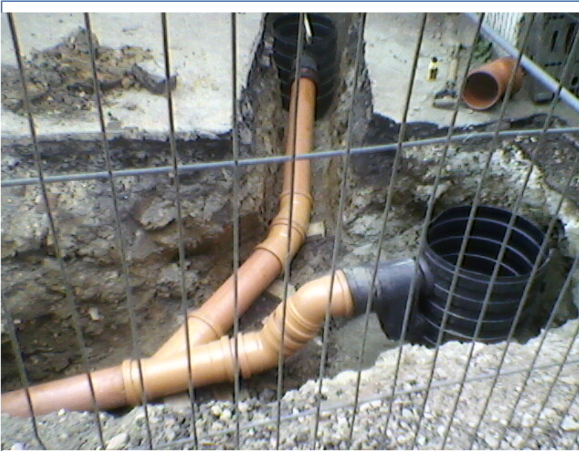
Shallow trench dug to expose gully pots
