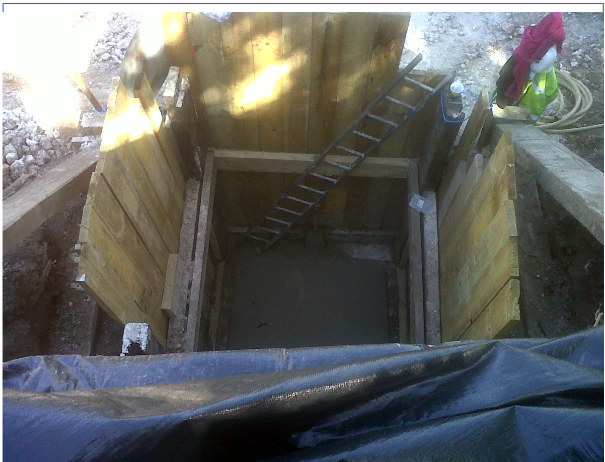
Service shaft with crash deck
