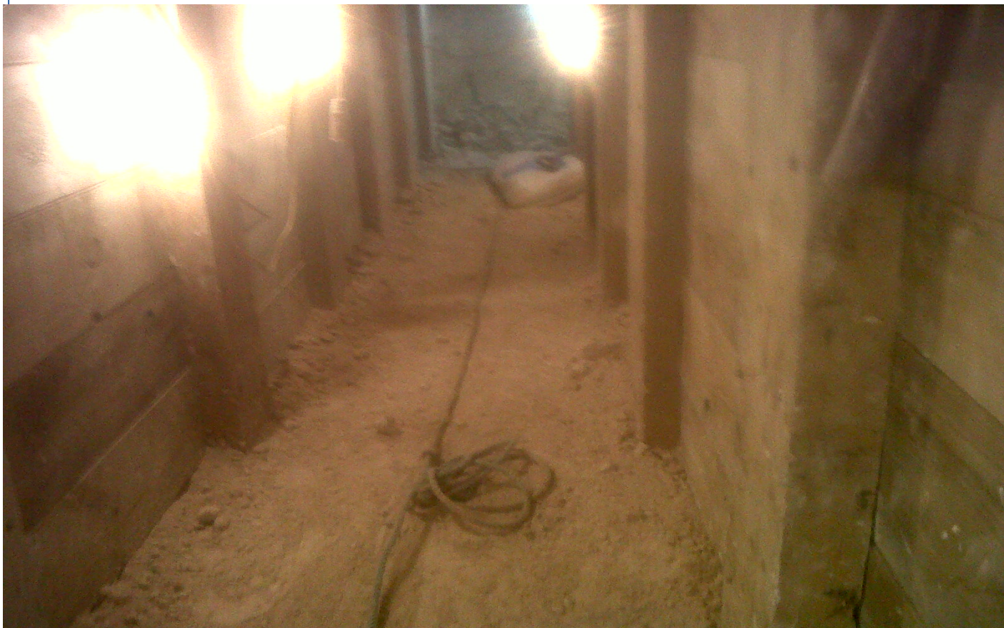
Tunnel formed to access main sewer
